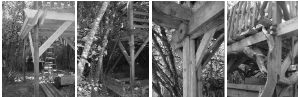
Image 1: Four very different ways to support a storage loft
