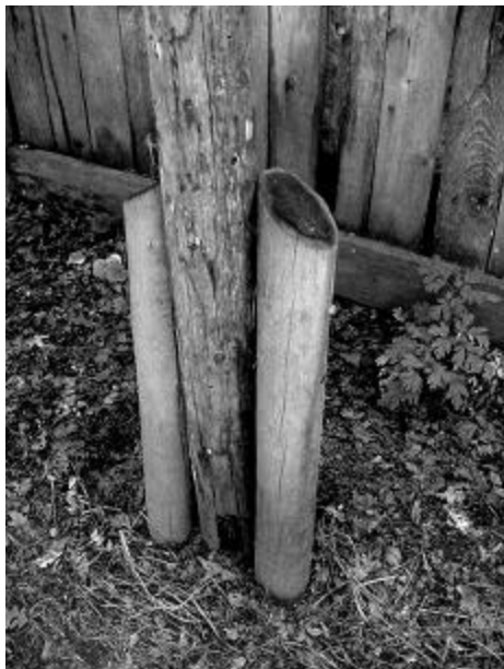
Sistering rotten support post. Note different approaches to through-bolting
