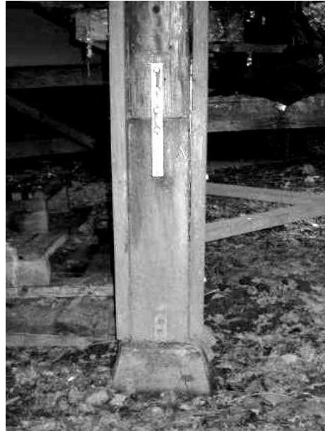
Sistering rotten support post. Note different approaches to through-bolting
