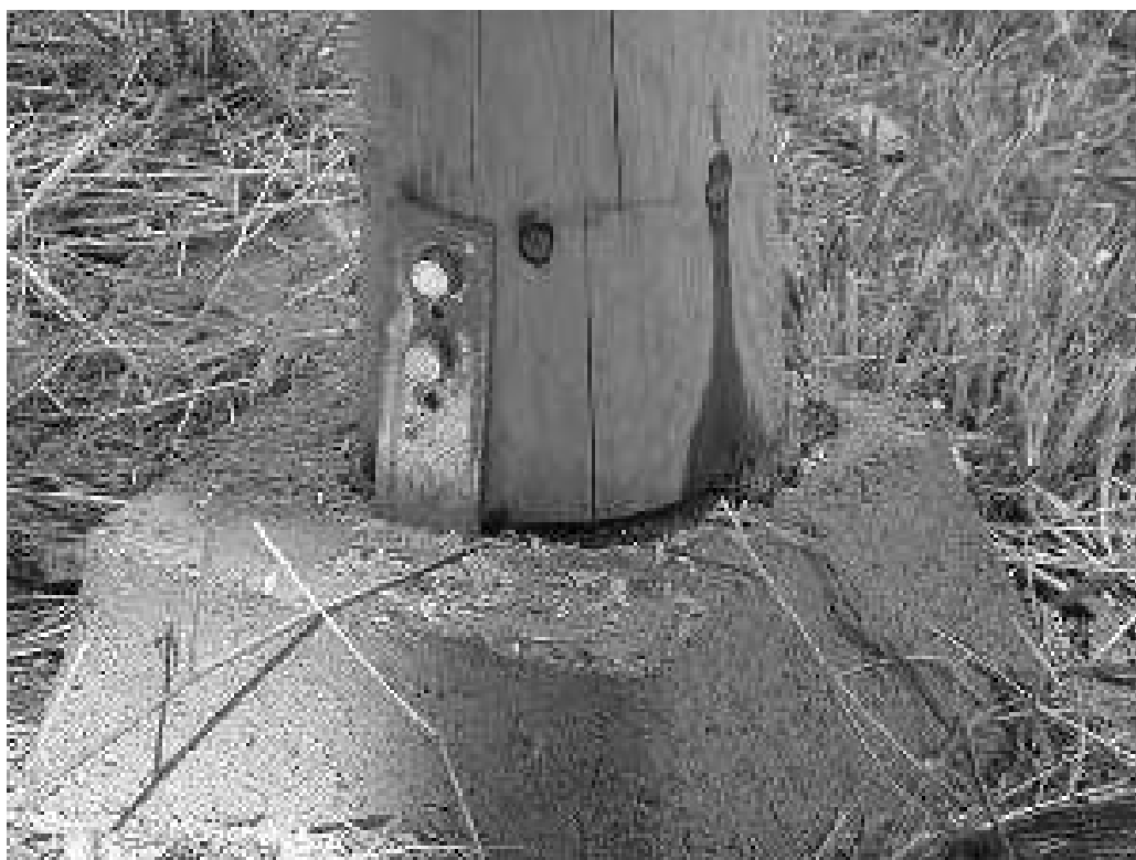
Figure 7 Post to pier pad attachment details
